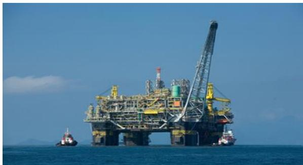
**Fig No: 1. Oil platform P-51 off the Brazilian coast is a semi-submersible platform. EPA handout 2009.**
